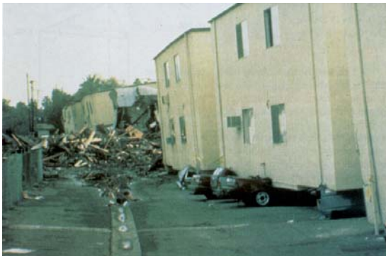
Soft-story apartment collapse in Northridge earthquake
