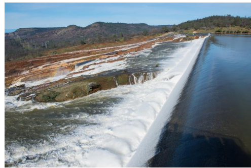
The Oroville Dam overflowing onto the emergency spillway on February 12. Image via Wikipedia.
