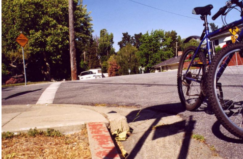
Creep on the Hayward fault evidenced by an offset sidewalk. Image via flickr.
